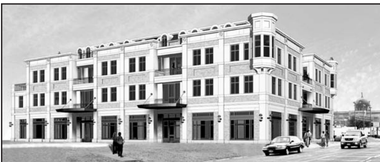
Phase 1 of Tamiro Plaza now under construction.
