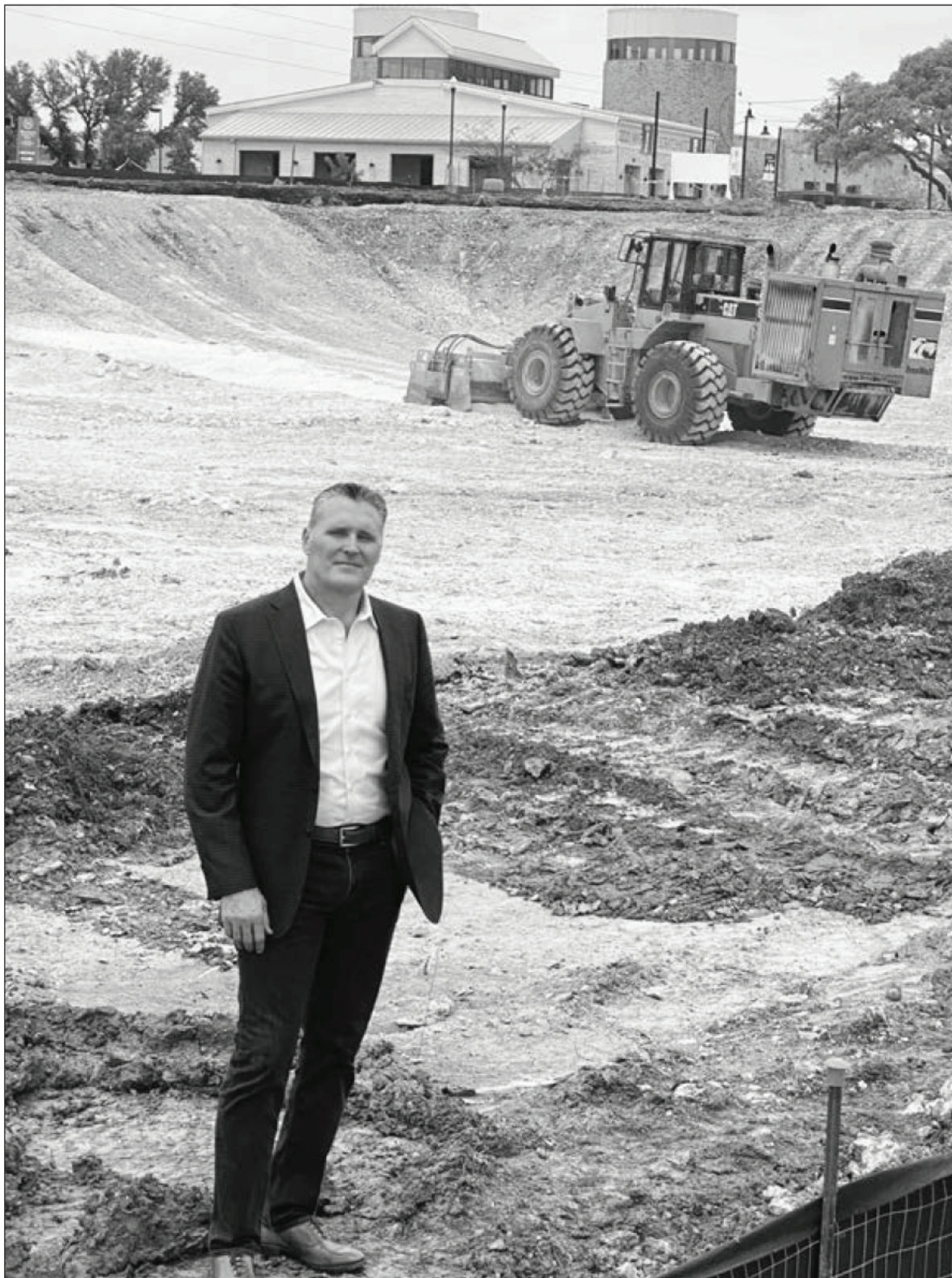
Jeff Novak of Novak Brothers is at the construction site for Summit Lofts in The Summit at Rivery Park.
